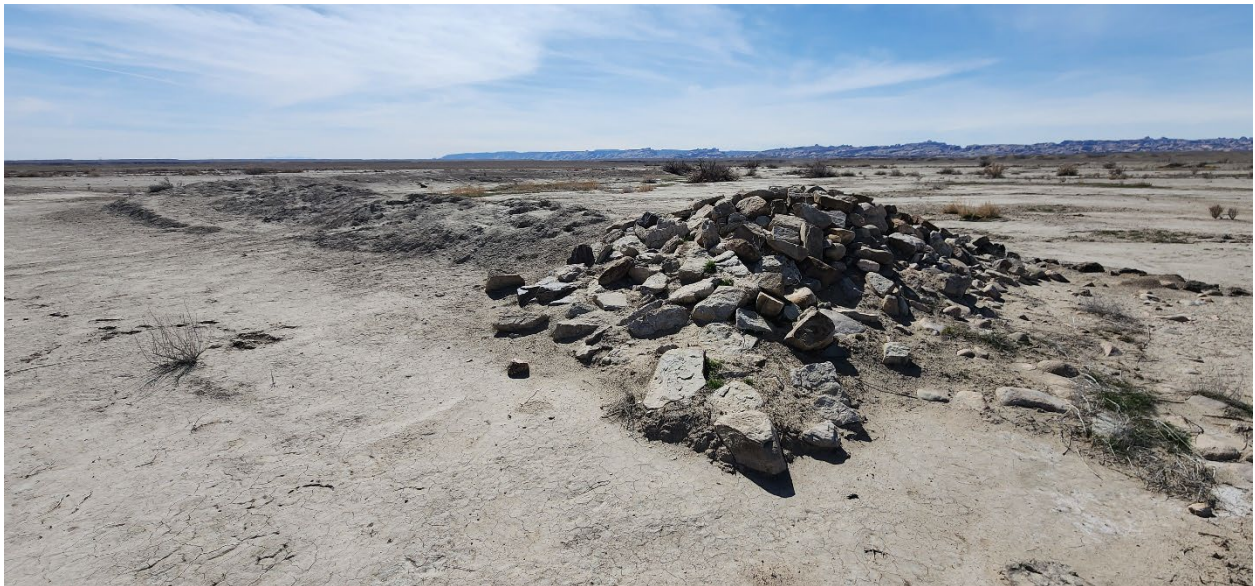
Photo 12: Looking southwest from northeast corner of the subject property, dike with rock shoring at end
