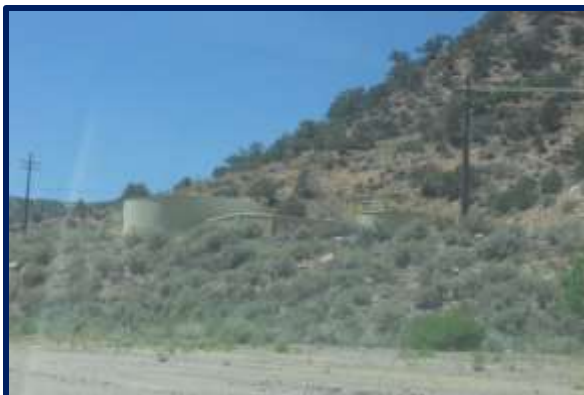
VIEW OF SUBJECT EXTERIOR
