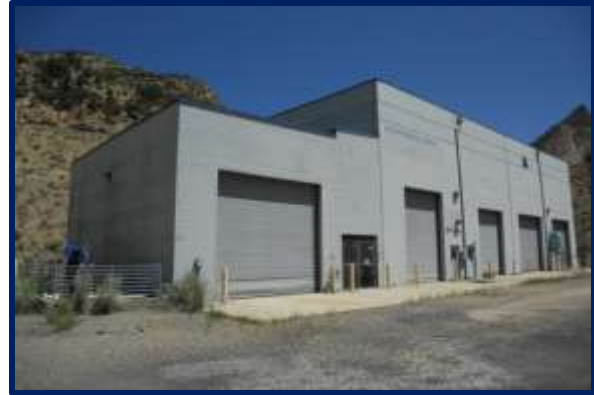
VIEW OF SUBJECT EXTERIOR
