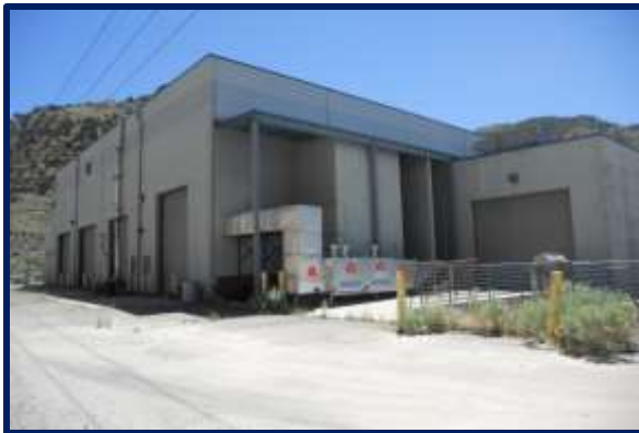
VIEW OF SUBJECT EXTERIOR
