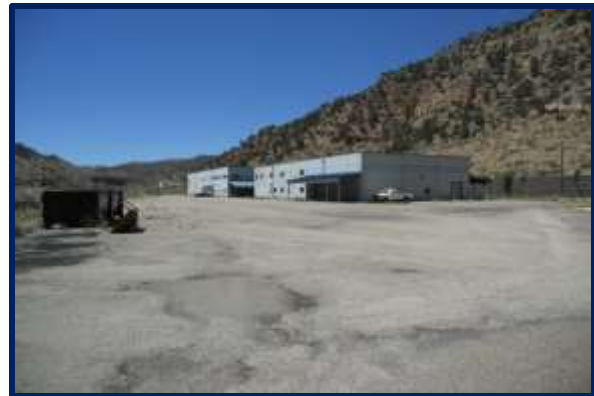
VIEW OF SUBJECT EXTERIOR
