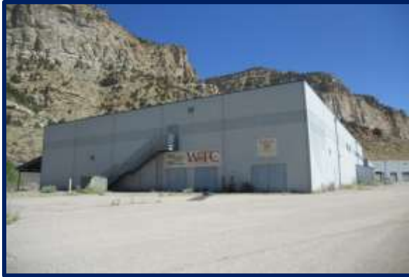
VIEW OF SUBJECT EXTERIOR
