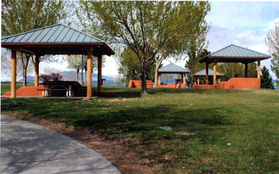
Picnic shelters along the Atkinville Wash.
